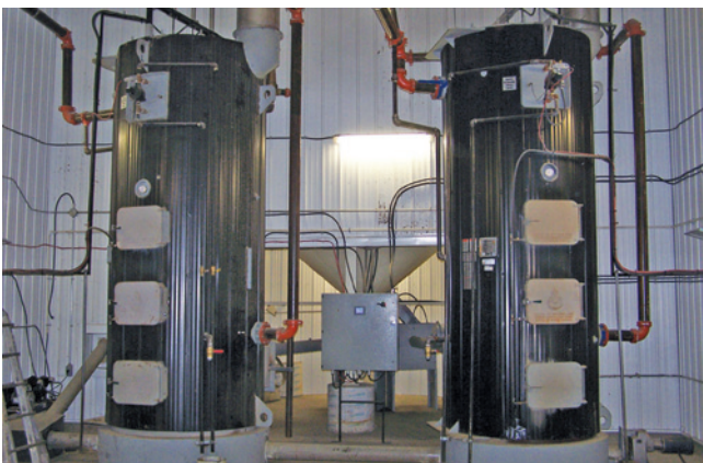
Commercial DBB Models Are Pressured Systems With BTU Ratings From 750,000 to 5.5 million BTUs
